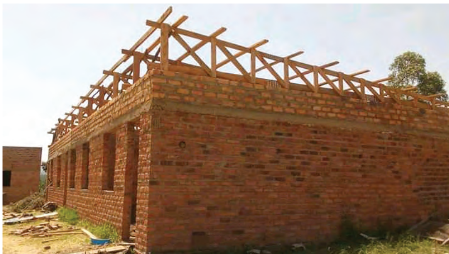
COVID-related shutdowns stalled construction at the Life School.
