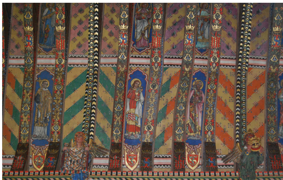
Nave Roof, St. Mary's, Huntingfield.
