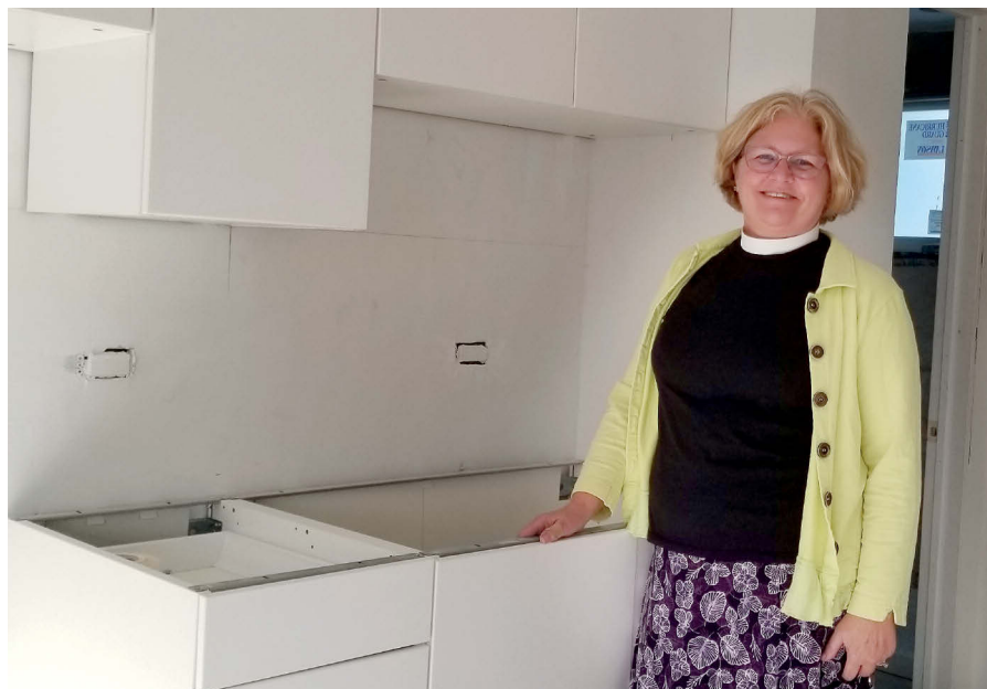
The Rev. Debra Maconaughey displays a kitchen under construction, where a hurricane left devastation. St. Columba photo
