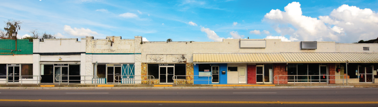
Abandoned storefronts in Williston, Florida, southwest of Gainesville
