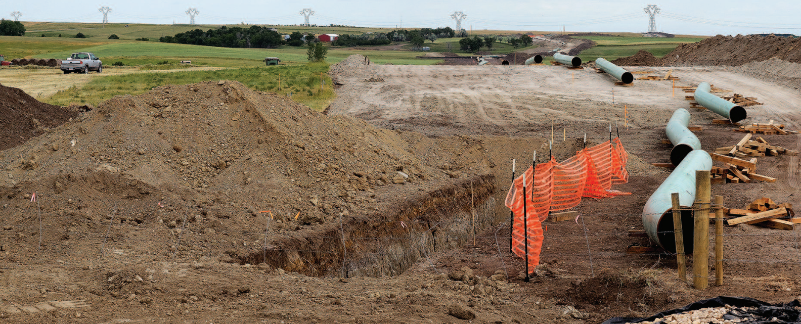
The Dakota Access Pipeline in the early stages of its construction
