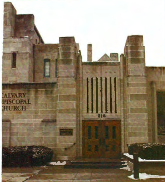
The entry to the Parish House at Calvary Church, Pittsburgh, was moved from its original relatively remote and inaccessible location (left) by using a basement window (center). The new entrance is more conveniently located at grade. (Photos courtesy of The Design Alliance Architects; photo at right by Ed Massery)
