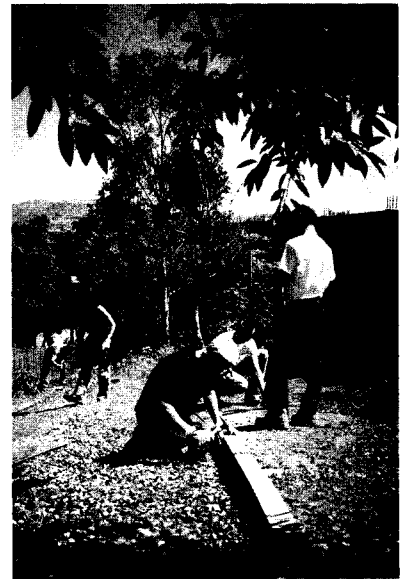
Volunteers de-rail salvaged lumber.
