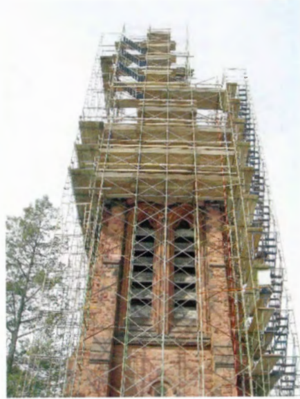
Scaffolding encloses the spire of Christ Church, Poughkeepsie, N.Y.
