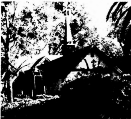
The chapel at St. Mary's Retreat House, Santa Barbara, Calif., which is owned by the Sisters of the Holy Nativity.
