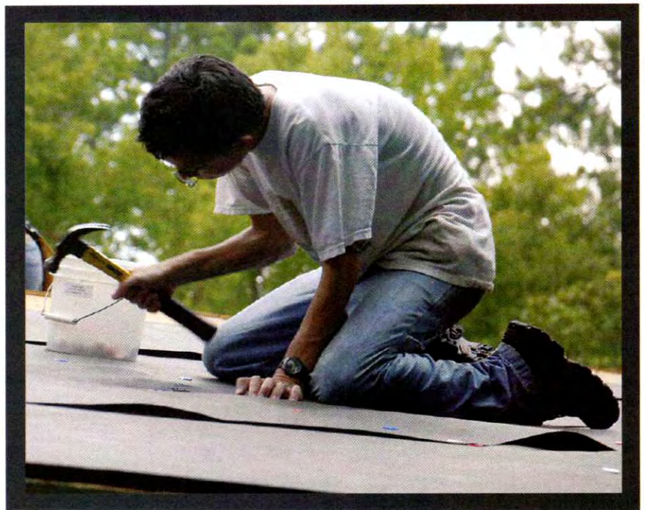
Roof repair in Summerville, S.C.
