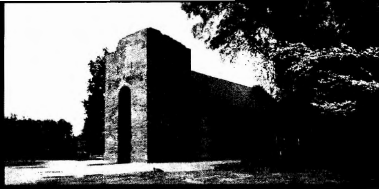
The bell tower, which is believed to date from the mid-17th century, is considered among the oldest structures in the United States. Reenactors come ashore on April 26. The historically accurate church was added to the restored bell tower in 1907.
