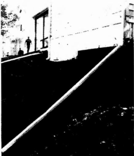
Grace Church, St. Marys, W. Va., lost most of its backyard to Hurricane Ivan's flood waters. It is now perilously close to a 60-foot drop to a creek. The Rev. Richard Heller, rector, said engineers have told the parish the rest of the bank could erode during the next six weeks. Representatives of FEMA, the Army Corps of Engineers, and interested citizens met to discuss plans and funding to prevent further slipping in the historic area.
