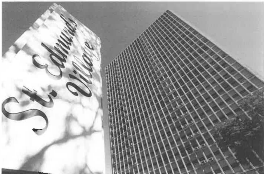
Below: After years of disrepair, the renovated apartment building on South Michigan Avenue in Chicago is full with a waiting list of more than 200 applicants.
