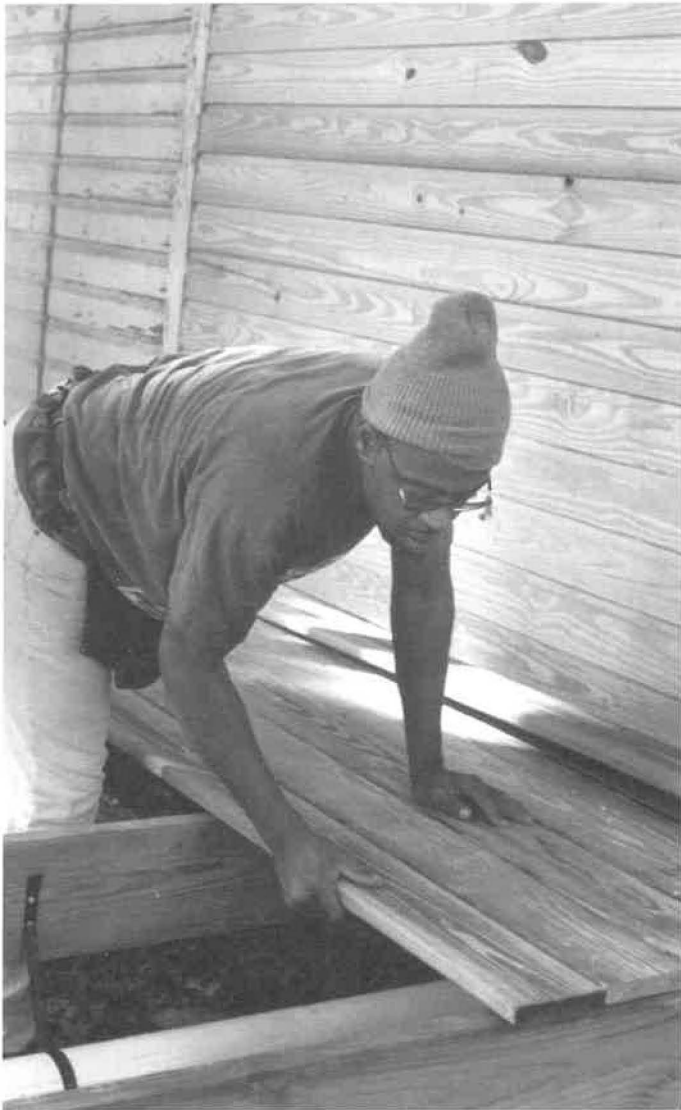
Operation New Hope carpenter-in-training fits floorboards for a porch.
