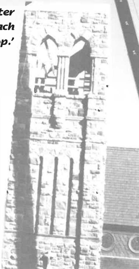
“When the structural work on the tower began,” Mr. Kampfe said, “major problems were found. The mortar had turned to sand. The whole tower had to be taken down and rebuilt.” It was decided then to replace the original steeple. When the new 16-foot pyramid was raised with a crane, “It was a traffic-stopper,” long-time member Connie Oakes said. The oldest parishioner, 104-year-old Elmer Wheal, was there to watch. The cross-topped peak completes the symmetry of the building.
