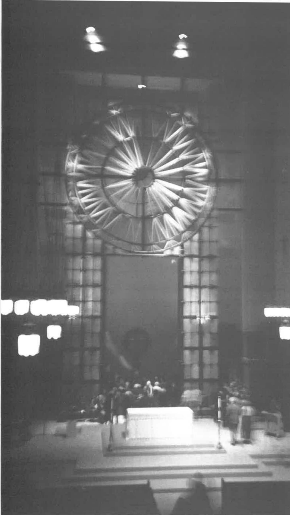
Remodeled Cathedral: A festival Evensong was held recently at St. Mark's Cathedral in Seattle to dedicate the remodeled west wall of the 70-year-old building. The $3.5 million project includes a glass screen behind the altar stretching 57 feet from floor to ceiling, with a circle near the top. When the central panels of the altar screen are opened, they reveal a chapel containing several historic mementos, including a tall Celtic cross originally atop the roof.
