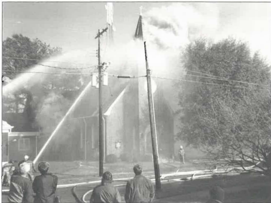
Church of the Advent, Enfield, N.C., was damaged heavily in this 1993 fire.
