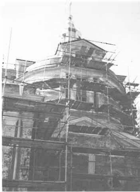
Repair work to St. Nikolai Orthodox Church.
