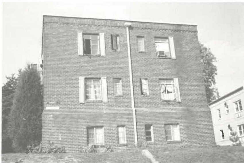
An apartment building being renovated by CLI and its supporters.
