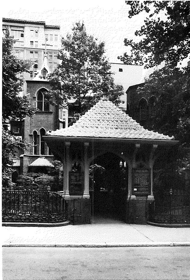
Church of the Transfiguration, New York City, also known as The Little Church Around the Corner.
