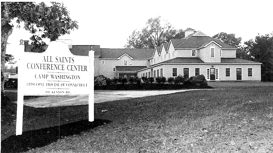
Renovated facilities at conference center in Lakeside, Conn.
