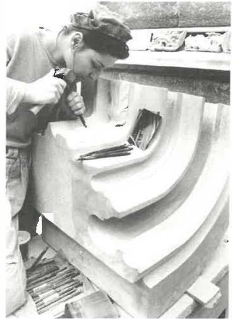
Therese Robb, a carver on the staff of Cathedral Stoneworks, chisels the finishing touches on a stone that is to be fitted in place on the renovated facade of the Jewish Museum in New York City, which is undergoing a $24 million expansion project. The Cathedral of St. John the Divine is donating to the museum a $5,000 stone pinnacle to crown the expansion project. [ENS photo by Mary Bloom]
