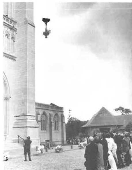
The finial stone is lifted to its place at Washington Cathedral. [Photo © 1990 Morton Broffman]
