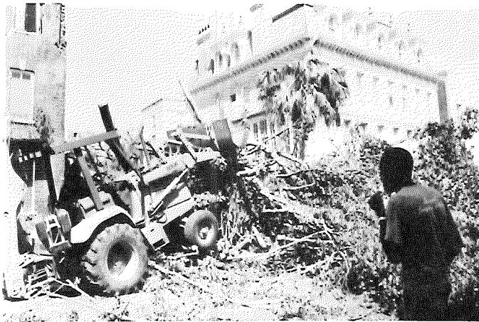
Clearing away rubble in Charleston, S.C., after Hurricane Hugo.
