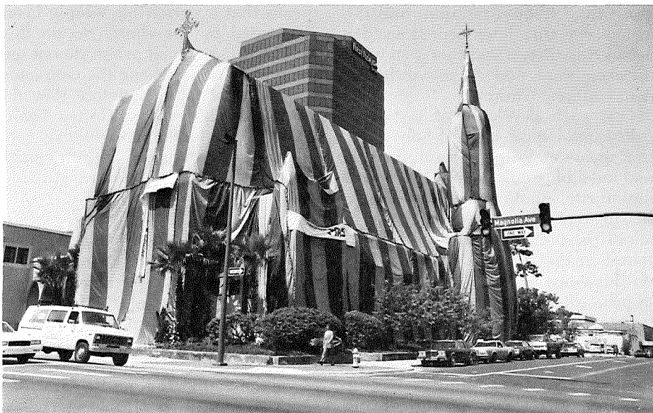
The Cathedral Church of St. Luke in Orlando, Fla. was tented from toes to tower last month as exterminators worked to rid the building of dry wood termites. It took over 20 hours and two tons of material to ready the cathedral for the fumigation.
