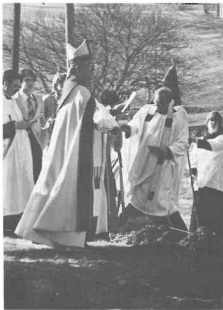
Bishop Ashby sprinkles holy water on the site of the new dining hall for St. Francis Boys' Home.
