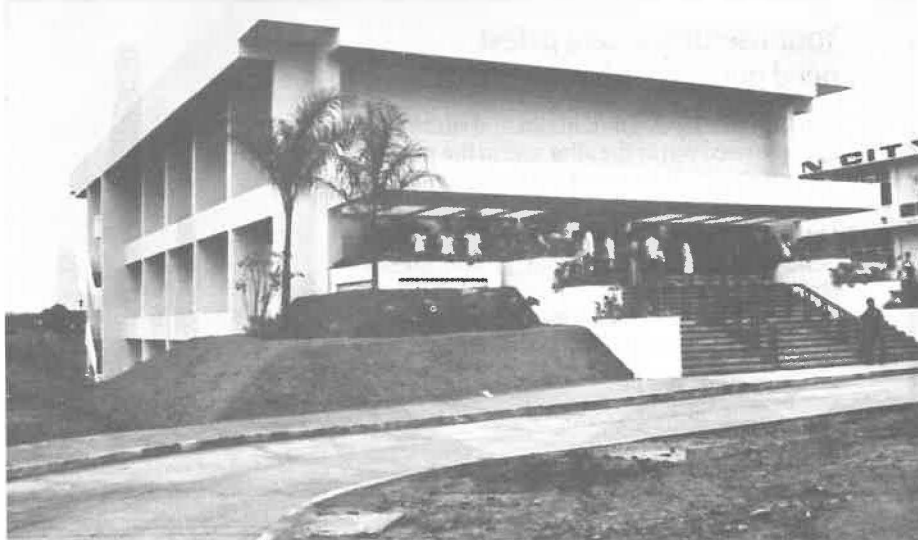
Wayland S. Mandell Hall, a new three-story library building, was completed on the campus of Trinity College, Quezon City, the Philippines. The building is named after the first president of the college's board of trustees, distinguished American priest and missionary, and dean of St. Andrew's for many years.
