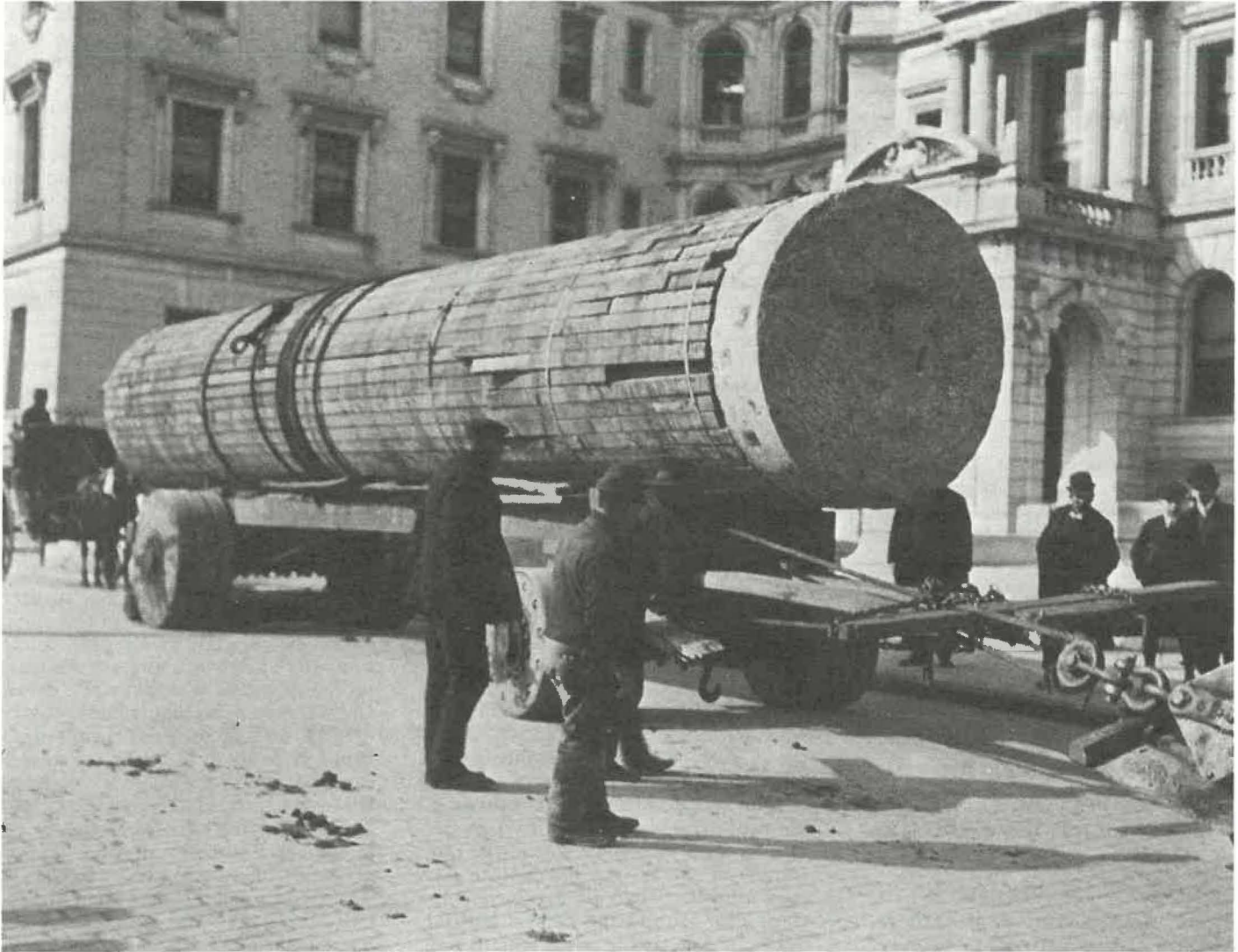
A column section for the Cathedral of St. John the Divine, New York City, turning into the cathedral close in 1903: And every manhole cover broke [see p. 8].
