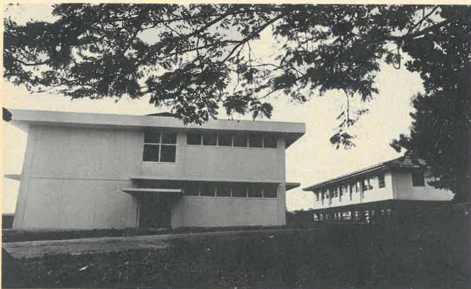
The new Science Building (left), and the Administration Building, a former dormitory.
