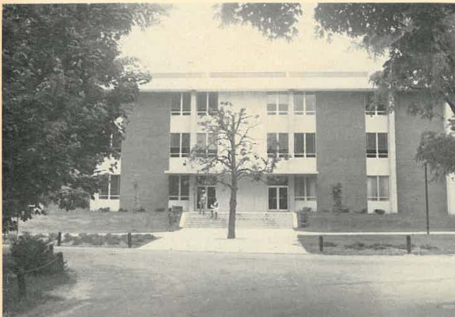
A new four-story classroom building has been completed.
