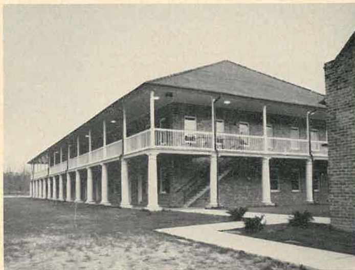
A TWO-STORY CLASSROOM and administrative structure, a combination auditorium-lunch room, and a headmaster's rectory, all constructed in Louisiana Colonial style, were dedicated in February at the New Episcopal High School, Baton Rouge, La. Situated on a 47-acre tract in suburban Baton Rouge, the school has been operational at that location since last September, and has a current enrollment of 262.
