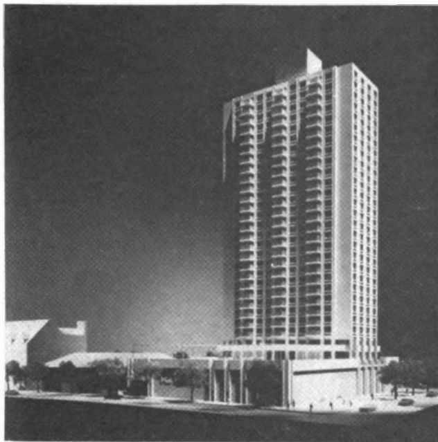
Trinity School and Apartments
