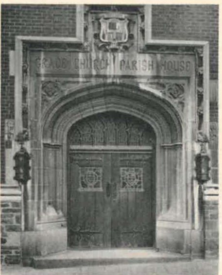
ENTRANCE TO GRACE CHURCH PARISH HOUSE UTICA, NEW YORK
