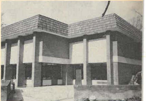
LOWER: Sinclair Hall newly constructed in Alexandria
