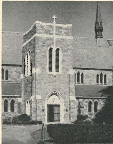
CATHEDRAL CHURCH OF ST. LUKE PORTLAND, MAINE
