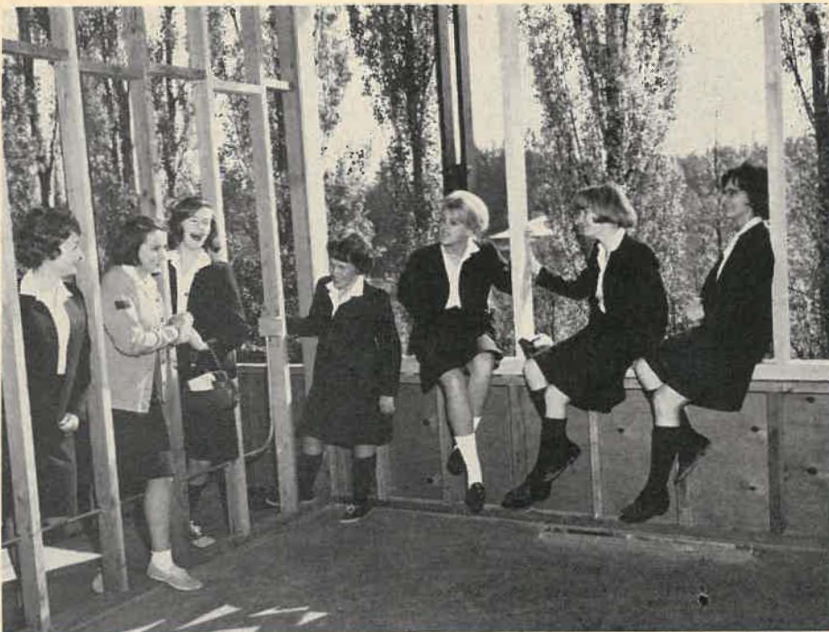
St. Helen's Hall students pause at dormitory being constructed on new 32-acre campus.
