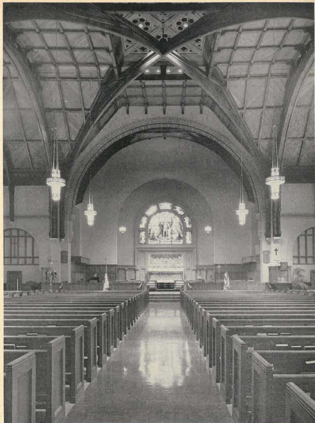
Interior of the newly restored St. Michael and All Angels'. The church was rededicated in May of this year.
