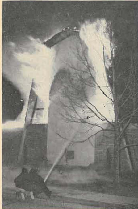
Our Saviour, Pasco, Wash.: Damaged beyond salvation.
