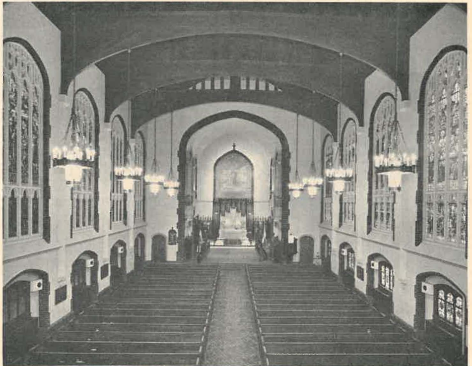
The air conditioning system in the 55-year-old St. Luke's Church, Atlanta, utilizes existing hot air ducts, with outlets under each ground level window, to supply conditioned air from a 60-ton capacity unit in the basement. Warm air, being lighter, is allowed to remain below the high ceiling.
