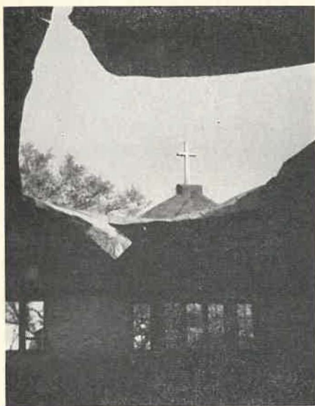
Parish Hall, St. Paul's, Savannah
