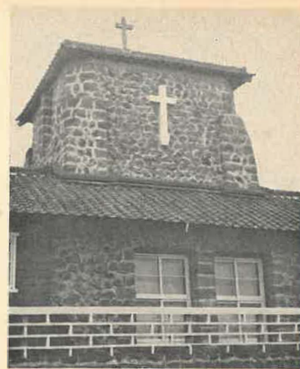
St. Andrew's at KEEP, before typhoon. The church was one of a number of KEEP buildings damaged by the storm.
