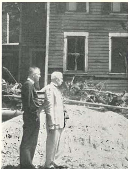
BISHOP HATCH , suffragan of Connecticut surveyed hurricane damage, found that many Churchpeople had sustained extensive property damage, such as this wrecked house belonging to a parishioner of Trinity Church, Seymour, Conn. With the Bishop is the Rev. Harold Edwards, rector of Trinity Church.
