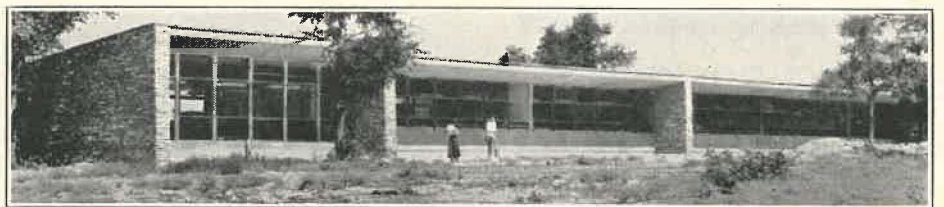
CLASSROOM building, new St. Stephen's, Austin.
