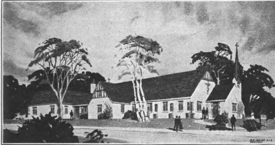
¶ The above sketch shows the proposed building for St. David's Church, Cambria Heights, L. I., N. Y., in the English Gothic style. The nave contains 150 pews, with exposed trusses overhead, and a rector's study and parish hall are included in the rear. The exterior walls will be built of economical cinder blocks, finished with a warm, buff-colored stucco. The buttresses and corner quoins will be reddish brick, which will harmonize with the red tiles of the roof.
