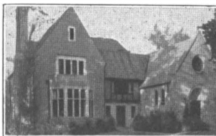
ST. FRANCIS HOUSE, MADISON, WIS.
