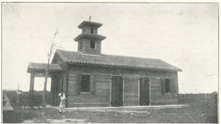
Large doors are an important feature of this new church building in Vertientes, Cuba. They provide added ventilation and make it possible for overflow crowds to sit outside the church on hot summer nights and hear the sermon. The new building has been sponsored by Graham H. Bienvenu, manager of the sugar central; it was designed by the Ven. John H. Townsend, Cuban archdeacon and LIVING CHURCH correspondent.
