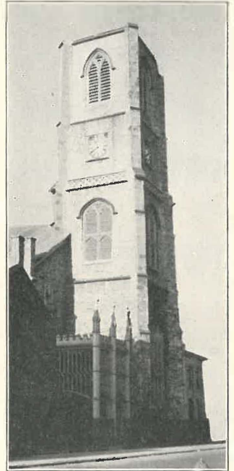
"CHRISTMAS CHURCH": Its ceiling is likely to fall.
