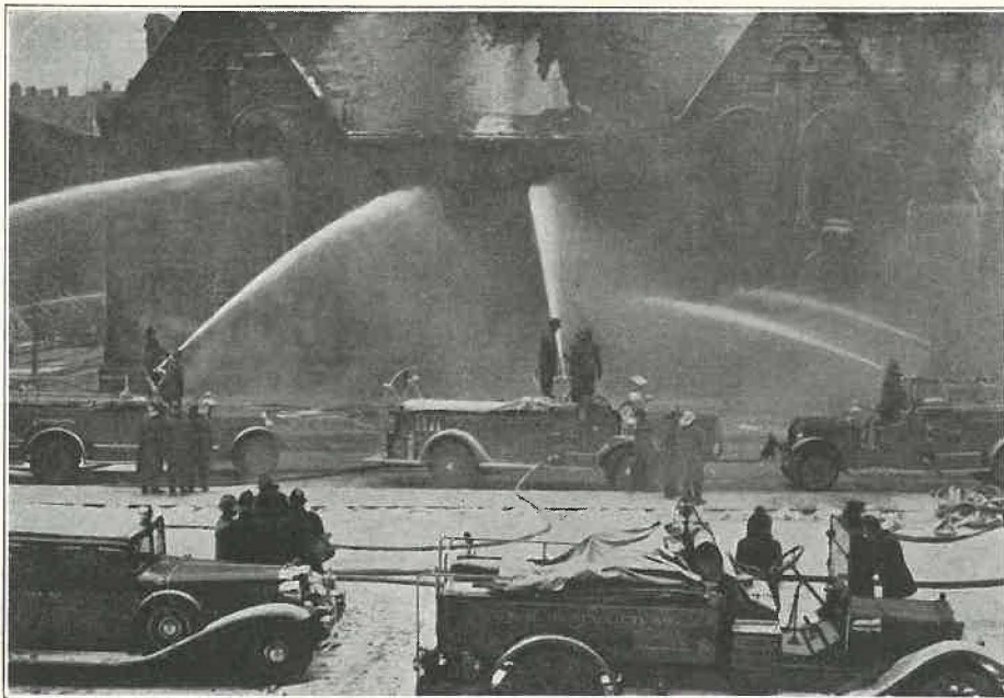
FOUR-ALARM FIRE AT ST. MARTIN'S, NEW YORK CITY
