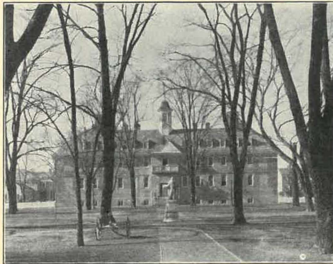
WREN BUILDING, COLLEGE OF WILLIAM AND MARY The oldest academic building in the United States
