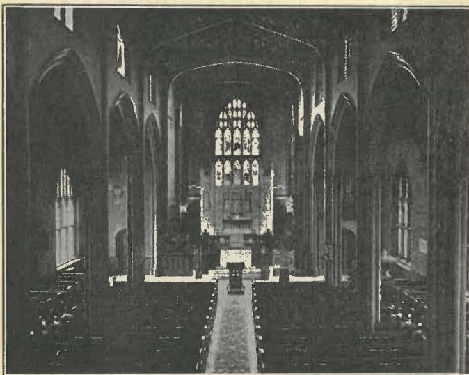
INTERIOR BEFORE THE FIRE
